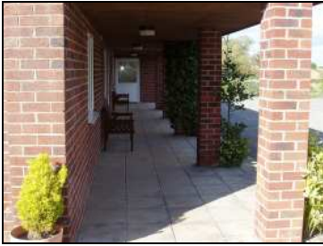
Covered walkway access to front doors Cottages 2 & 3 from the car park
